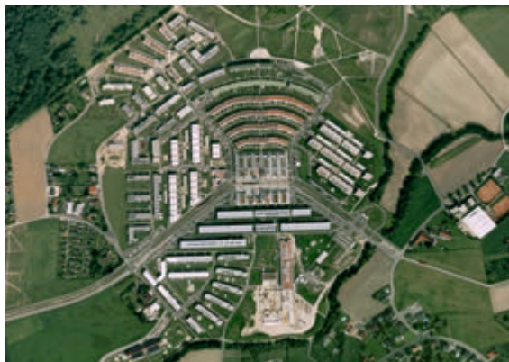
■ obr. 34_Solar City Linz – Pichling
