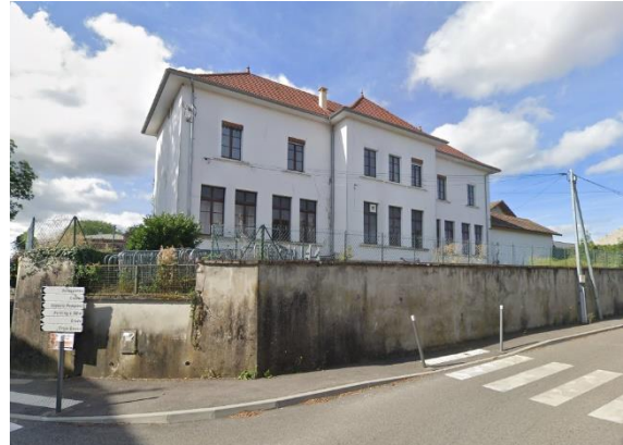
Figure 2: Goole image of the building to renovate in the village of Chimilin
