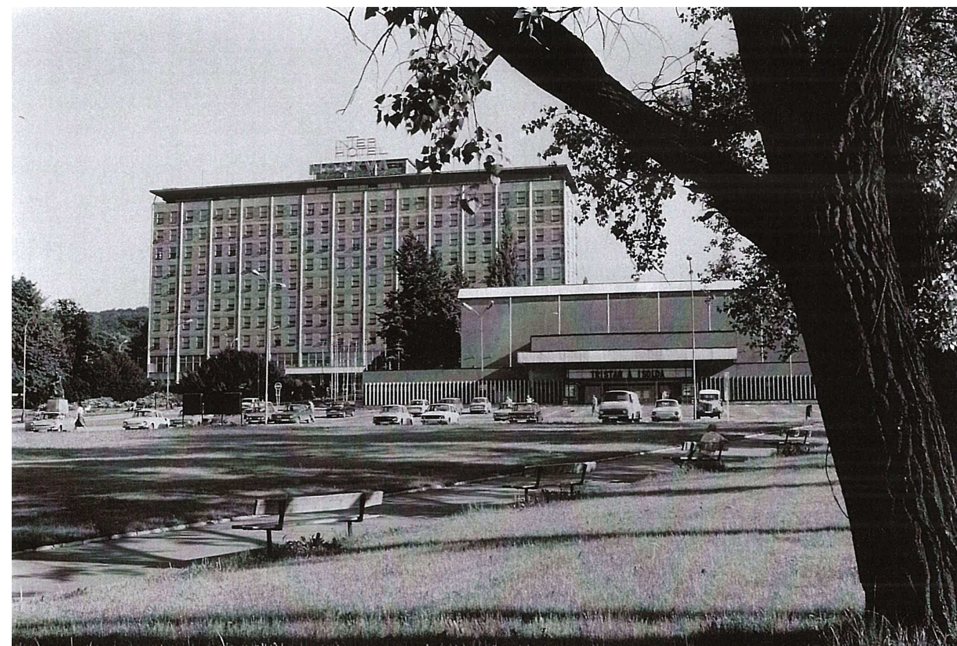
The Great Cinema facade and the Interhotel Moskva. Exterior of the cinema after treatment of the facade by spraying with dark green resin Teraplast. Source: MMZ, Kubik, 1983
